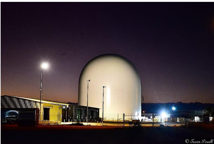
Second attempt at building a new inflatable cement Silo at 25 Berth (the first exploded).
