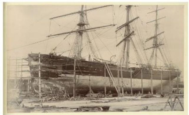
On Fletchers Slip Adelaide after undergoing repairs
